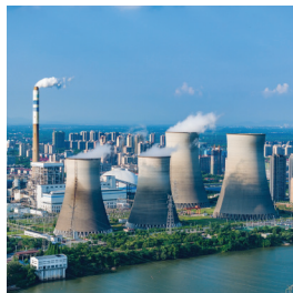
Thermal Power Plants
